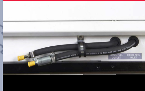
INPUT/OUTPUT FUEL PIPE
