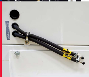
Fuel inlet and outlet
